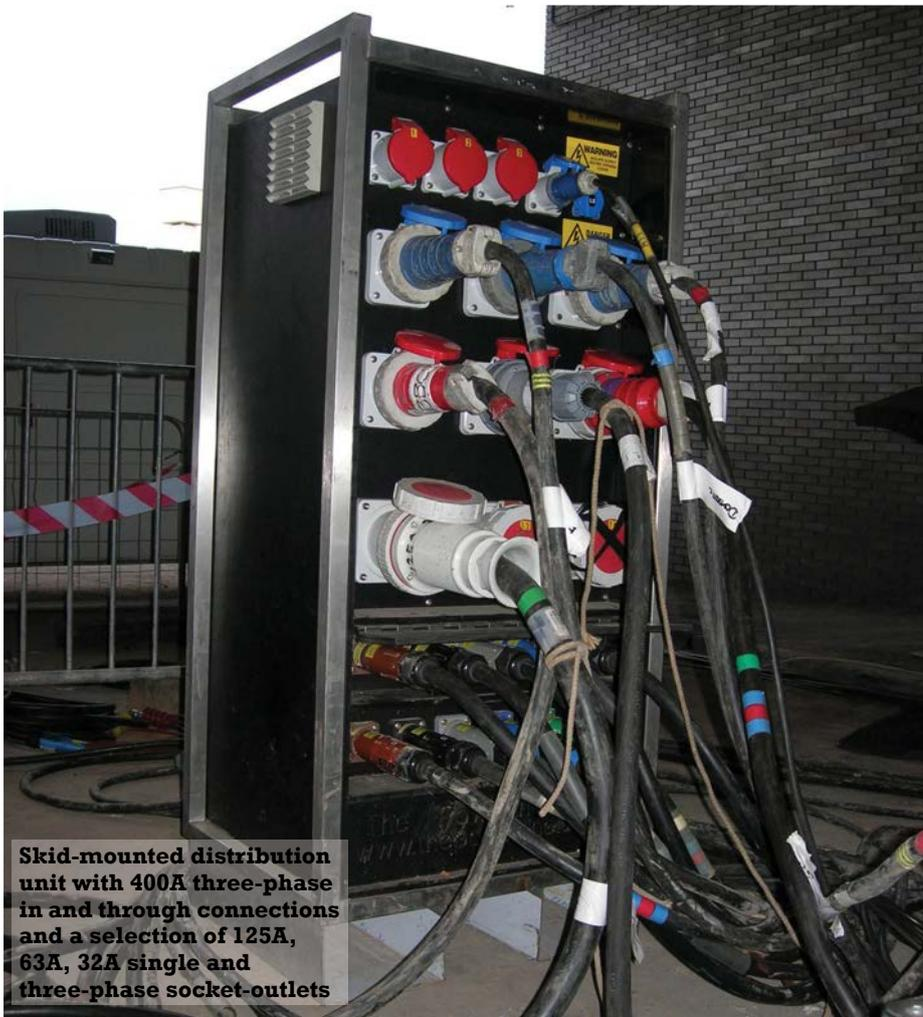
Skid-mounted distribution unit with 400A three-phase in and through connections and a selection of 125A, 63A, 32A single and three-phase socket-outlets
